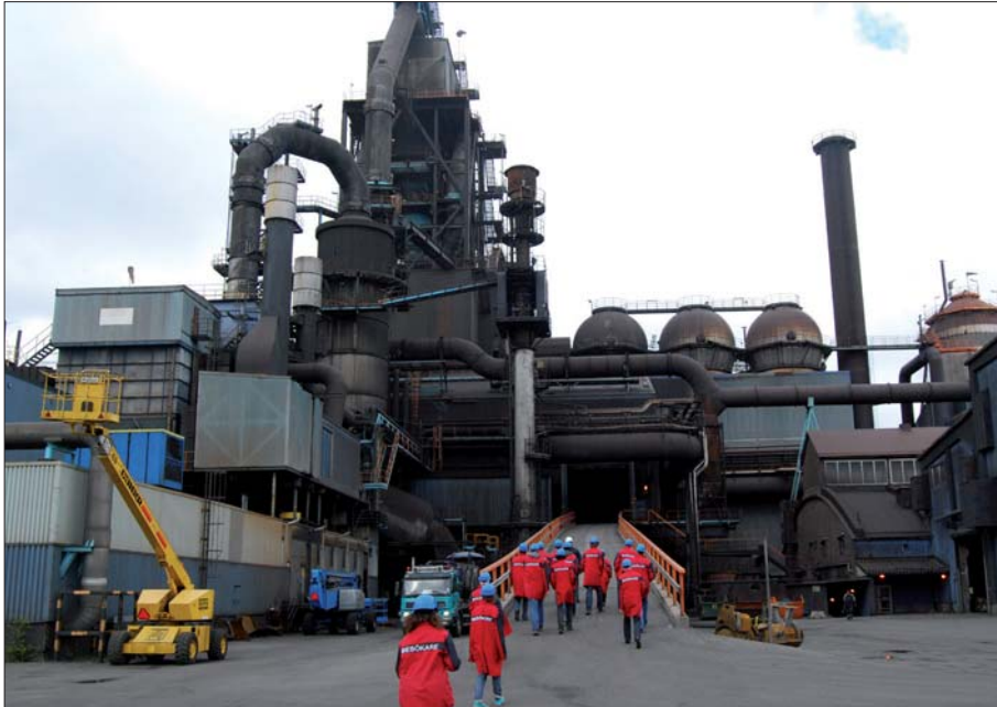
An optional excursion to SSAB was arranged. SSAB works with high strength steel and employs 8 700 people in over 45 countries. The participants visited the blast furnace and steel plant.
