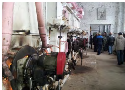
Figure Ko7.2. Mazut-burning municipal heating central in Kortkeross near Syktyvkar that can be converted to burning wood waste
